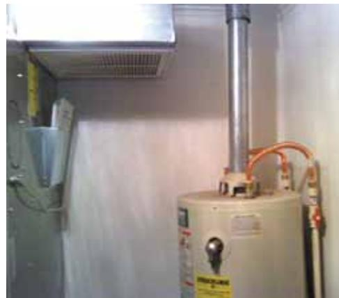
**The flue from a gas water heater near a return air vent can pose major health hazards.**
