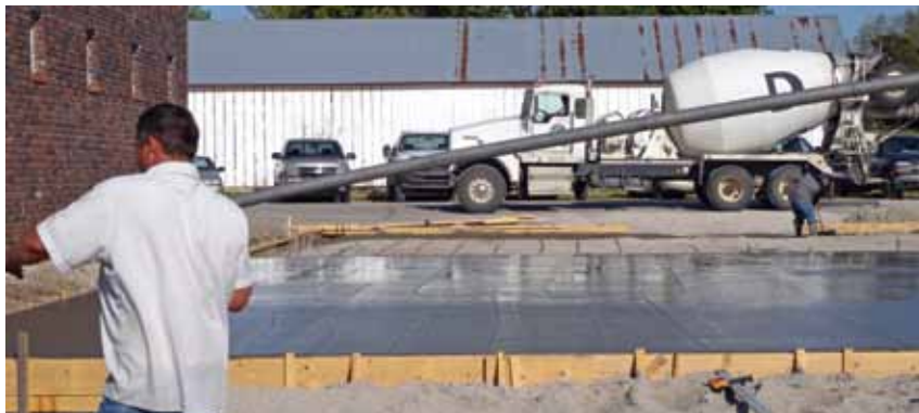
Crews spread a new foundation to Caney Valley's equipment warehouse.
