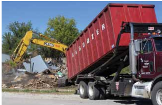
Dozers and trucks removed the rubble after demolition.
