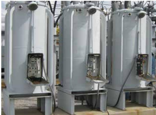
**These three voltage regulators were destroyed when a suspected metal thief cut a ground wire. Estimated cost for the lost equipment was \$75,000, but the salvage value was only a small fraction of that amount, hardly worth risking a life.**
