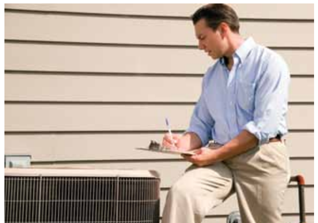
Air conditioner failures can be caused by a manufacturer's problem or an installer's mistake, but there's another cause you may not be aware of—restricted air flow.
