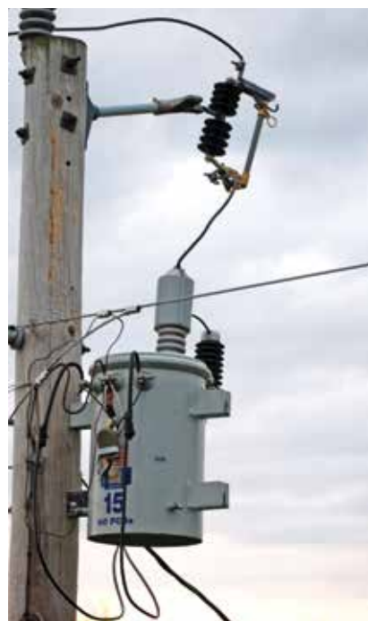
Transformers lower voltage to a level that's safe for use in your home. Homes served by electric co-ops can often be identified by transformers sporting redundant mounting brackets on the outside of the canister.
